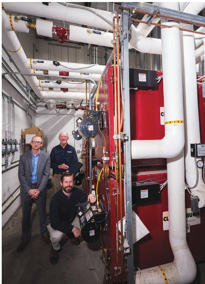
From left, Steve Knaub, Wayne Howe and Adam Shamenek pose next to Clean Burn CB500 boilers and below Bell & Gossett pumps.
